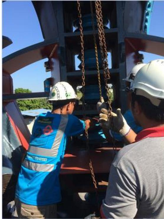
*Replacement of TBM cutter disc*
