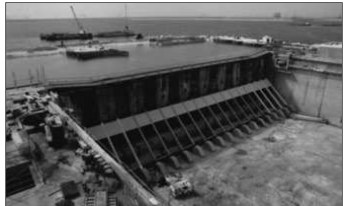
Figure 8: Dubai Dry Dock – dock gates
