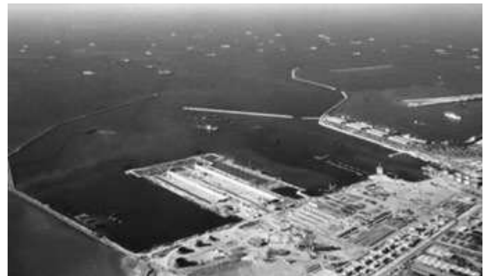
Figure 5: Dubai Dry Dock under construction
