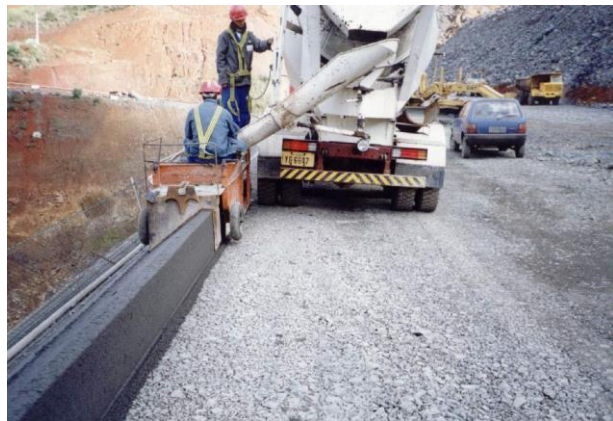
Extruded Curb Construction
