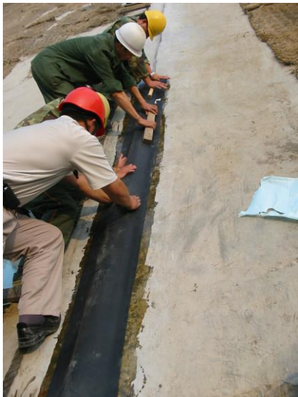
Plinth Construction (Itapebi Dam)
