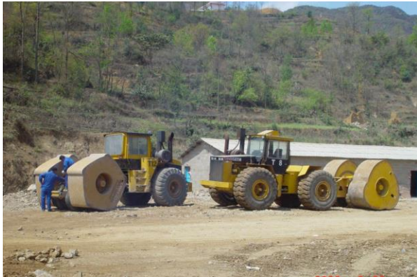
New Technology – Impact Compaction
