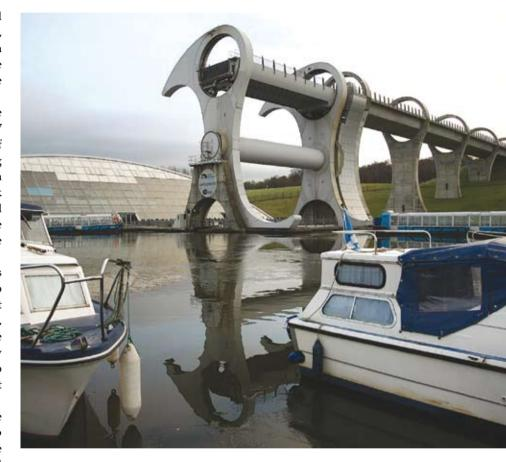
a dry well alongside the lower basin at the same time that a similar lower gondola is being raised by the opposite arm to the level of the aqueduct. Once released into the lower basin, the boats sail through a single lock and drop the final 3m to join the Forth and Clyde Canal.
