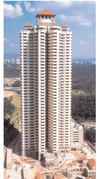
43 storey condominium in Mont'Kiara supported by G-Pile System.
