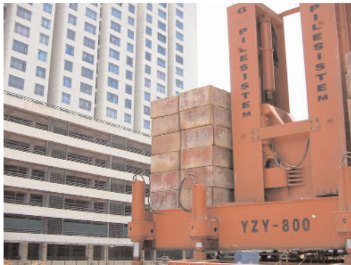
800 Tons Jacking Machine
