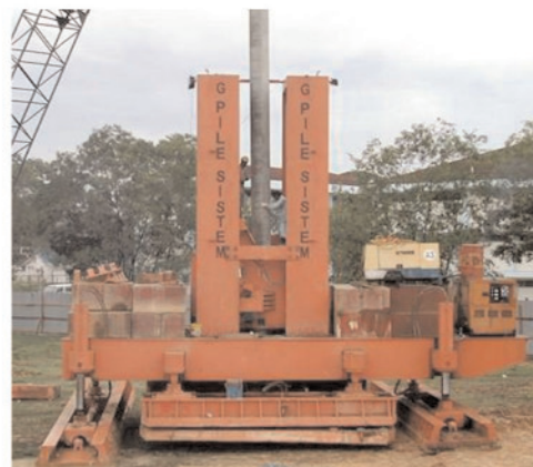
Pile jacking in progress
