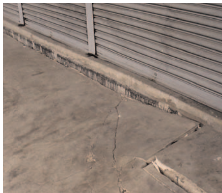
Figure 8 : Settlement of walkway and apron, common occurrence in soft ground such as marine soil
