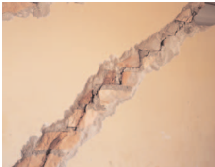
Figure 7 : Brickwall is highly sensitive to movements
