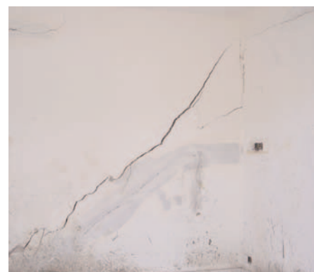
Figure 3 : Severe cracks due to differential settlement in the living room is not a welcomed sight
