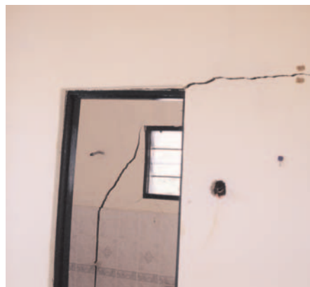
Figure 1 : Distortion of building due to excessive differential settlement
