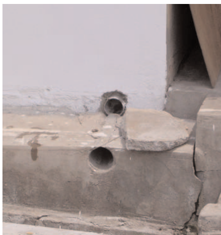
Figure 9 : Settlement of drain and services in soft soil
