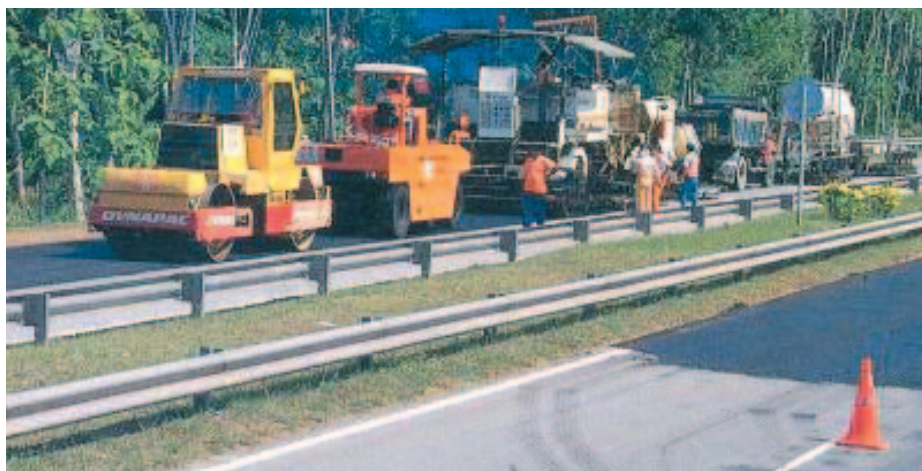
Figure 1: HIPR Equipment Train: Preheater, Remixer, Tipper, Rollers (Source: http://www.propel.com )
