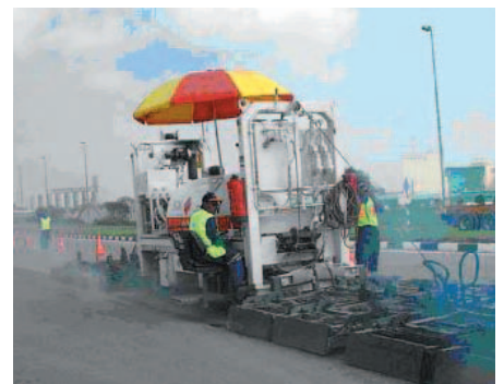
Figure 5: Heating the pavement surface with a preheater
