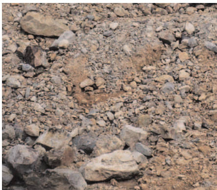
Figure 6 : Backfill indiscriminately filled with boulders can be a nightmare for foundation engineers
