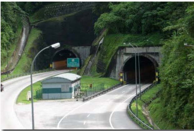
Karak Highway Twin Tunnel
