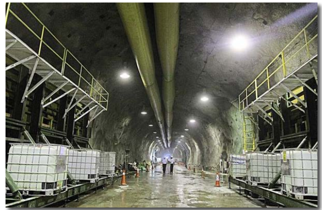
Sungai Selangor Water Transfer Tunnel
