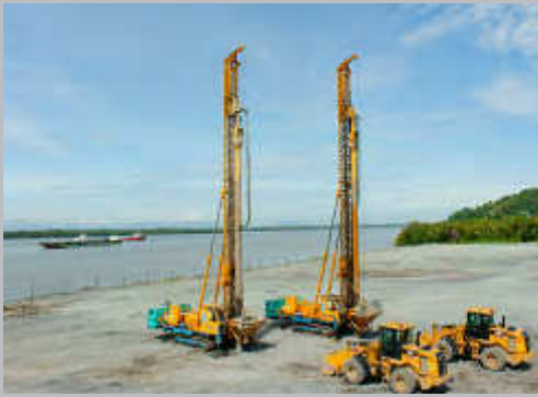
Vibro Stone Columns, Kuching
