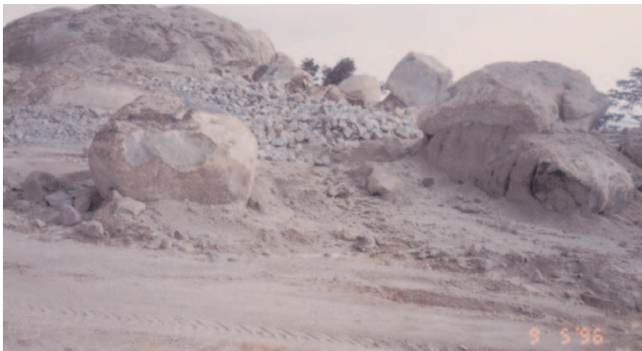
Blasting of outcrops and boulders
