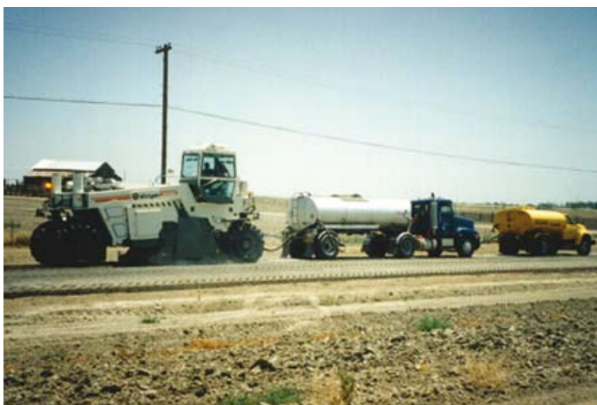
Figure 5: Cold in-situ recycling using foamed bitumen
