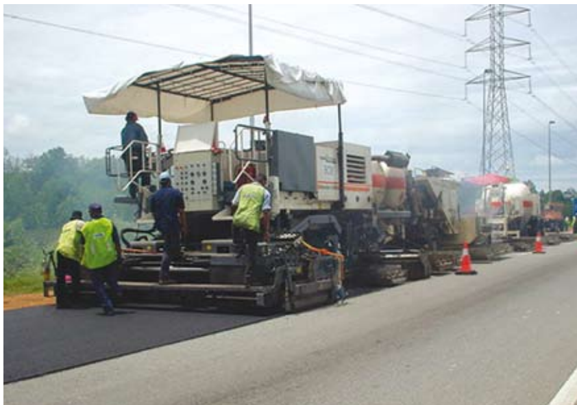
Figure 4: Hot in-situ recycling
