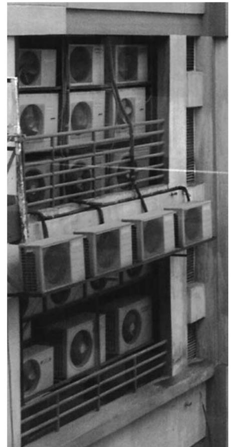
Figure 3: Typical air cooled split systems inadequately positioned in an architecturally challenged environment
