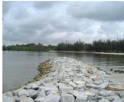
Figure 3: Revetment at Pantai Sri Cahaya (near Pulau Si Rusa)
