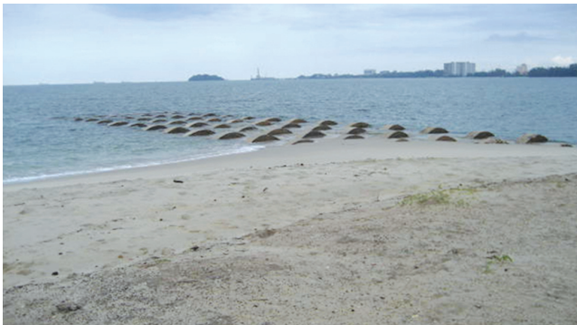
Figure 1: Bagan Pinang beach and drainage outfall
