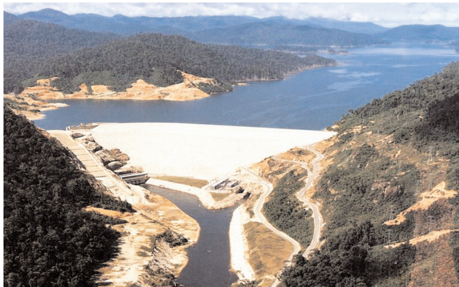
400MW Kenyir Hydropower Station in Terengganu
