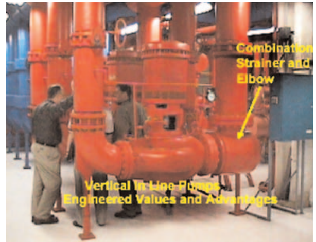
Figure 1: An installed VIL pump
