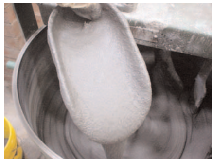
Figure 2: Mixing of reactive powder concrete with high workability
