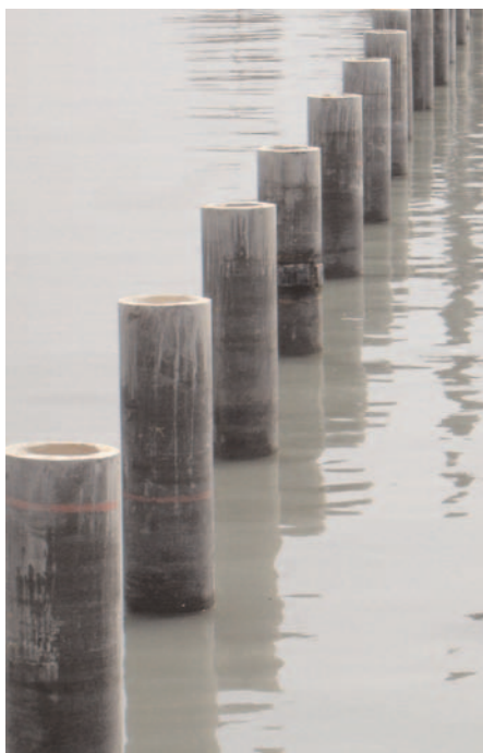
Figure 5 : Prestressed concrete spun piles driven in the sea
