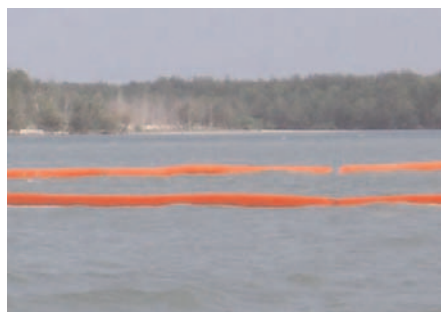
Figure 6: Silt curtain in use for environmental protection in coastal reclamation project
