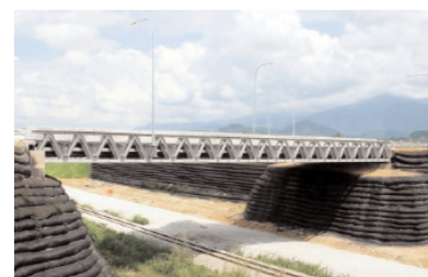
Geosynthetic reinforced bridge abutment
