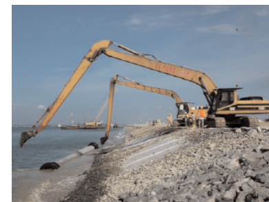
Launching of geosynthetic reinforcement on seabed
