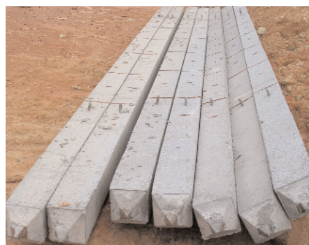
Figure 4: The present reinforced concrete piles of grade 45 N/mm 2
