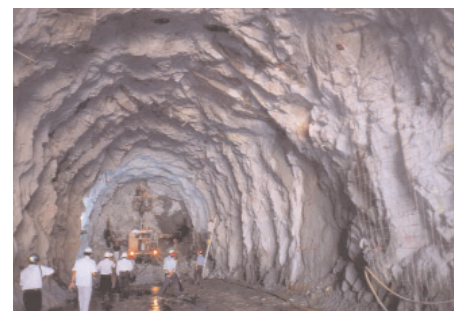
Tunnel in highly jointed granite - Sg. Selangor Dam diversion tunnel
