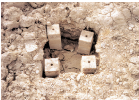
Figure 6 : Spacing of the piles are too close
