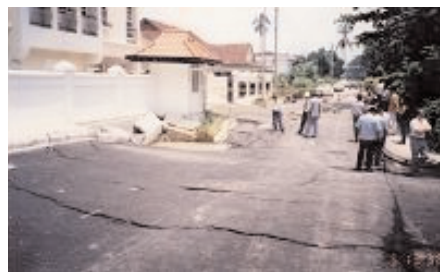
Figure 10: A sinkhole at Jalan Lidcole (GESB 1995)
