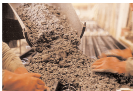
Figure 7 : No slump concrete used in vibrating formwork
