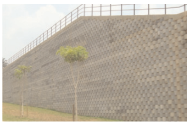
Geosynthetic reinforced segmental block wall
