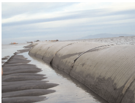
Figure 5: Geotube in use for coastal protection works
