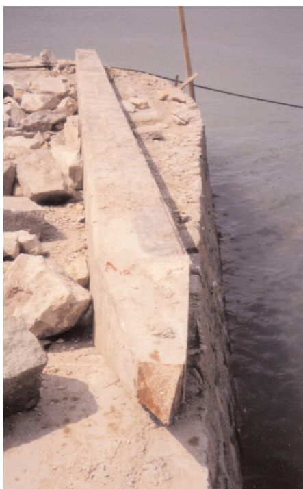
Figure 3 : Reinforced concrete pile used in the sea, not common these days
