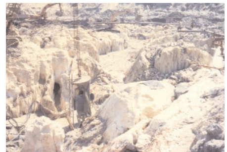
Limestone bedrock (highly pinnacled) vis-à-vis foundations - Kinta Valley
