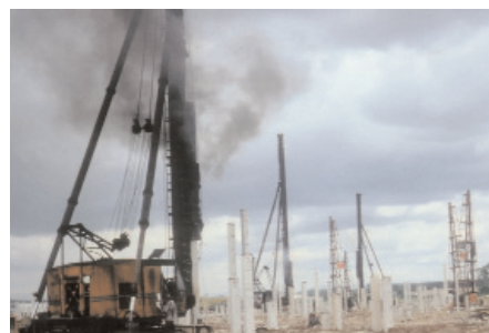
Figure 1: Diesel hammer, the old workhorse of the Piling Industry
