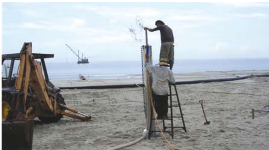
Figure 7: Installation of PEM system
