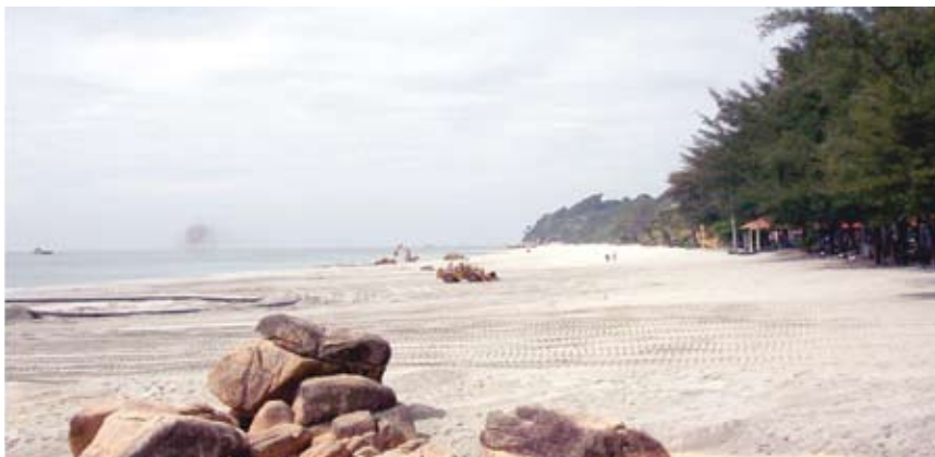
Figure 8: PEM system and sand nourishment at Teluk Cempedak completed in July 2004
